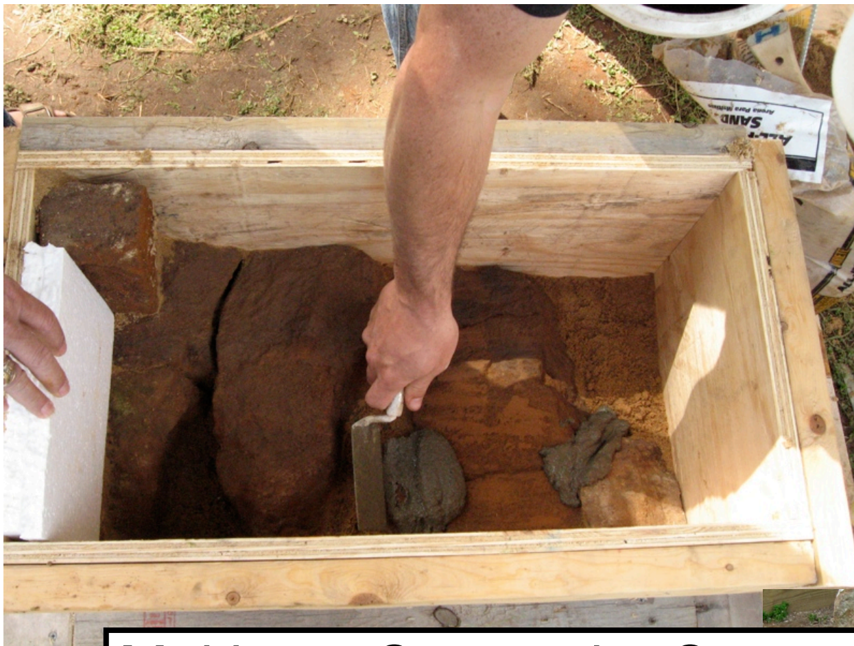
Making a Composite Cornerstone
