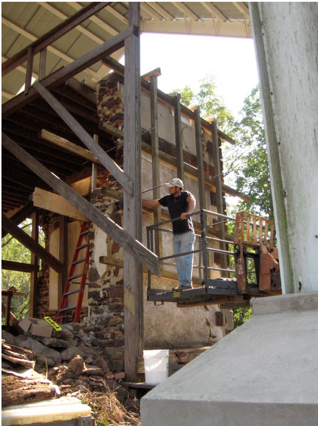
Strongbacks, tightened bolts, and a come-along
